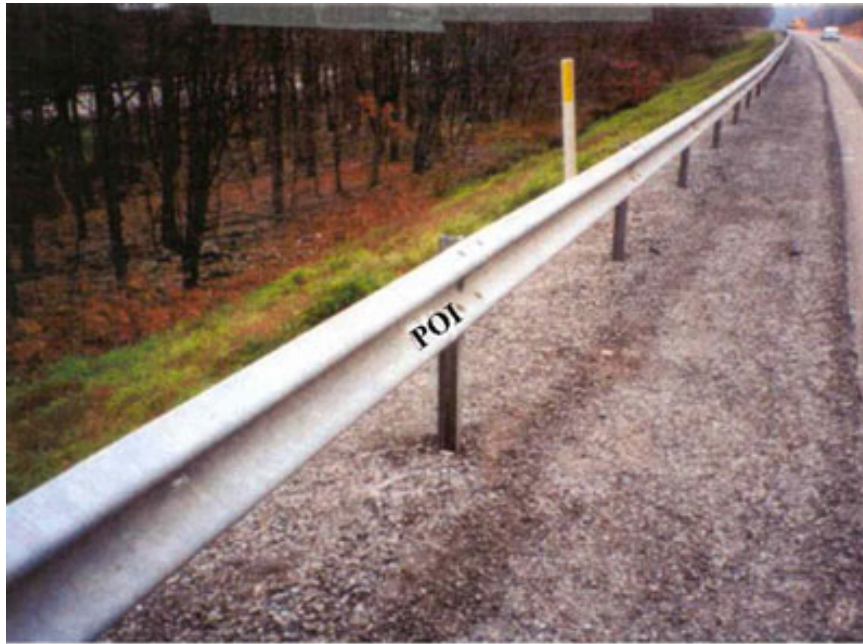
Photo 1. Guardrail on the South Shoulder of the Westbound Lane.
