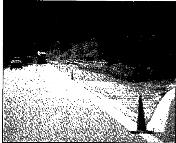
Figure 26. Coning for paint application
